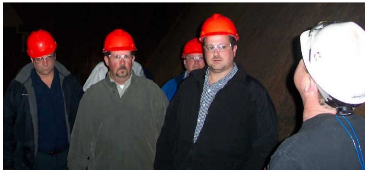
Right -- Tour participants had the opportunity to enter a Spurlock station unit boiler that was in shutdown mode that evening. Some of those who made the difficult entry via access door into the vast, dark boiler were Jay Adams, Doug Davis, Jim Brown and Chad Rausch, along with EKPC Engineering Manager and tour guide Jeff Schaefer (right).
